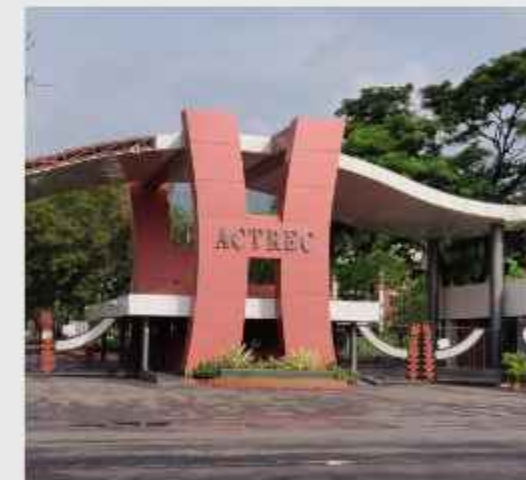
TATA MEMORIAL HOSPITAL: KHARGHAR, NAVI MUMBAI
